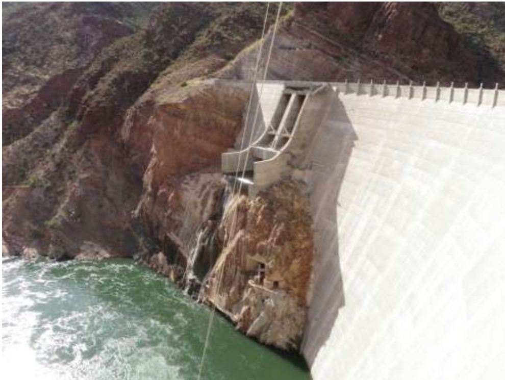
Figure 2 - Downstream view of Roosevelt Dam and right abutment spillway.
